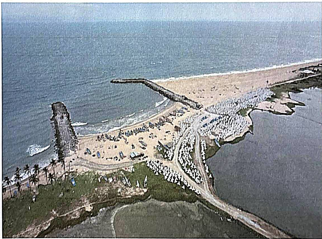
After Placing Breakwaters
